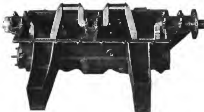
BEARINGS BOLTED TO UPPER HALF OF CRANKCASE.
